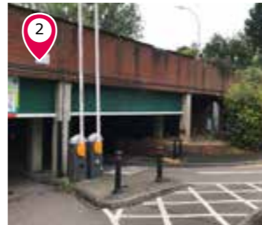
Water Gardens Car Park North
